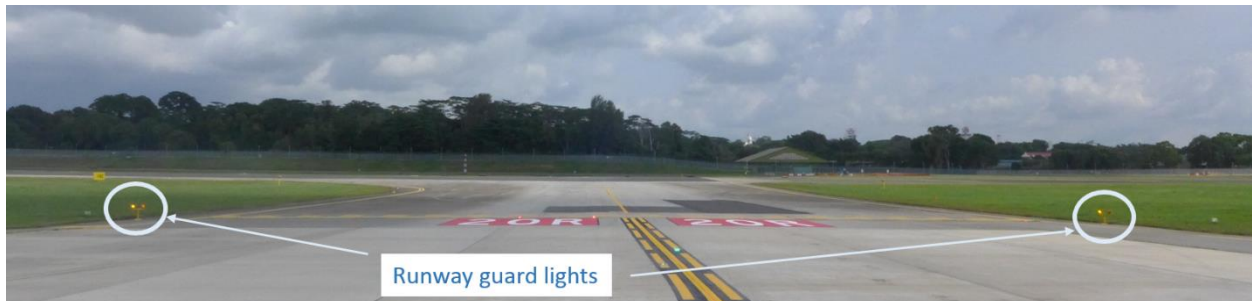
Figure 6. Runway guard lights at the side of a taxiway
