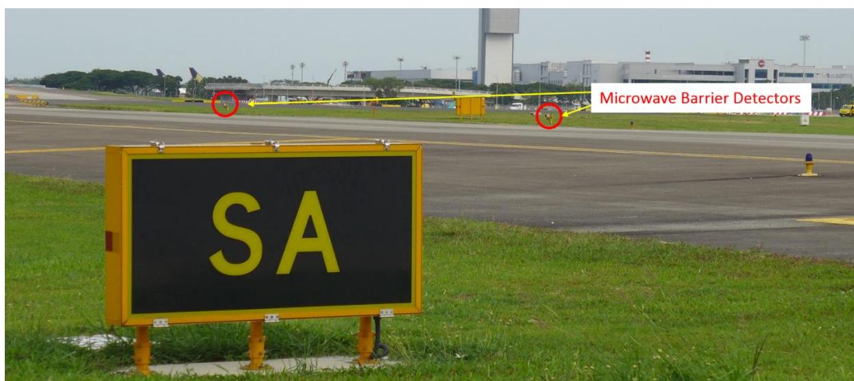
Figure 4. Microwave Barrier Detectors on Taxiway SA
