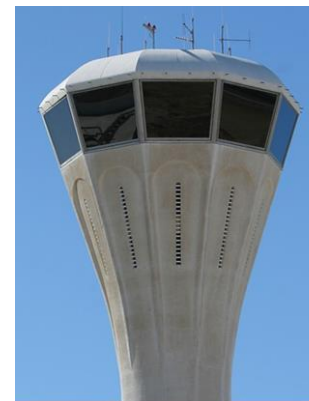
Figure 3. OMSJ Tower - visual control room
