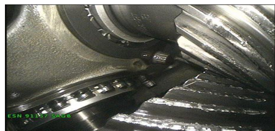
Figure 6. Damaged bevel gear
