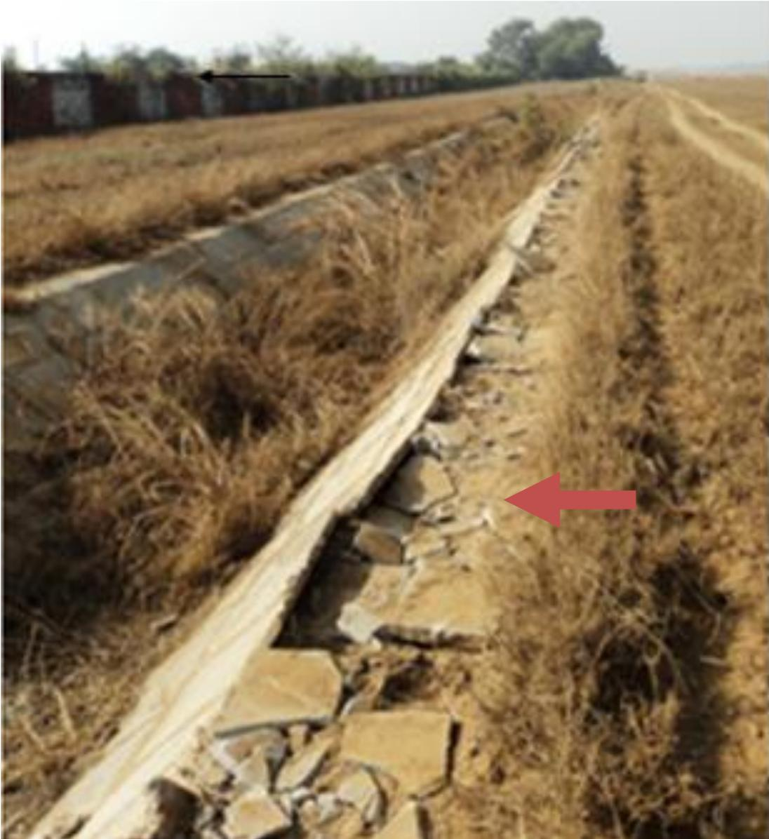
**Left main wheel rolled over the drain boundary area**
