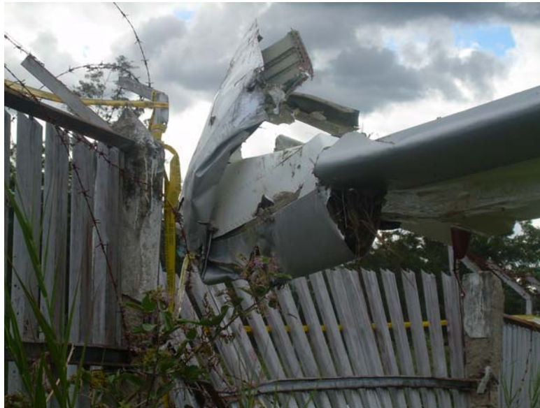
Figure 4: The aerodrome perimeter fence
