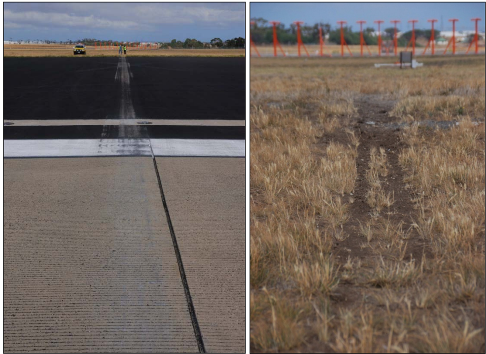
Figure 10: Typical contact marks on runway, stopway and grassed areas
