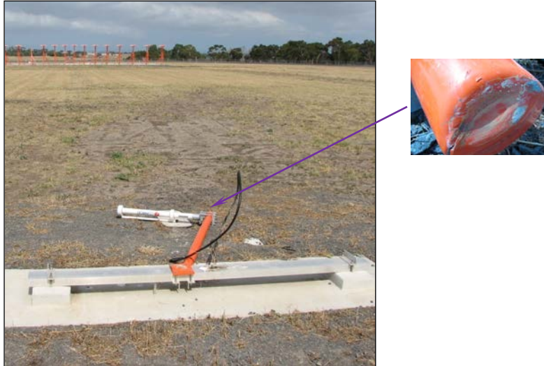
Figure 12: Localiser near-field monitor antenna
