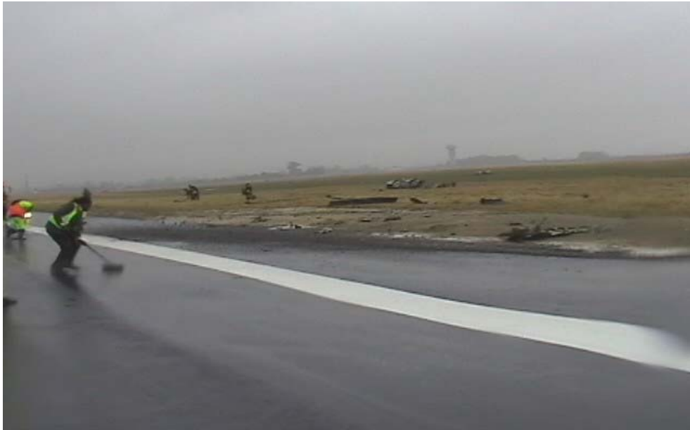
Photo 2: Showing the emergency personnel clearing debris from the runway.
