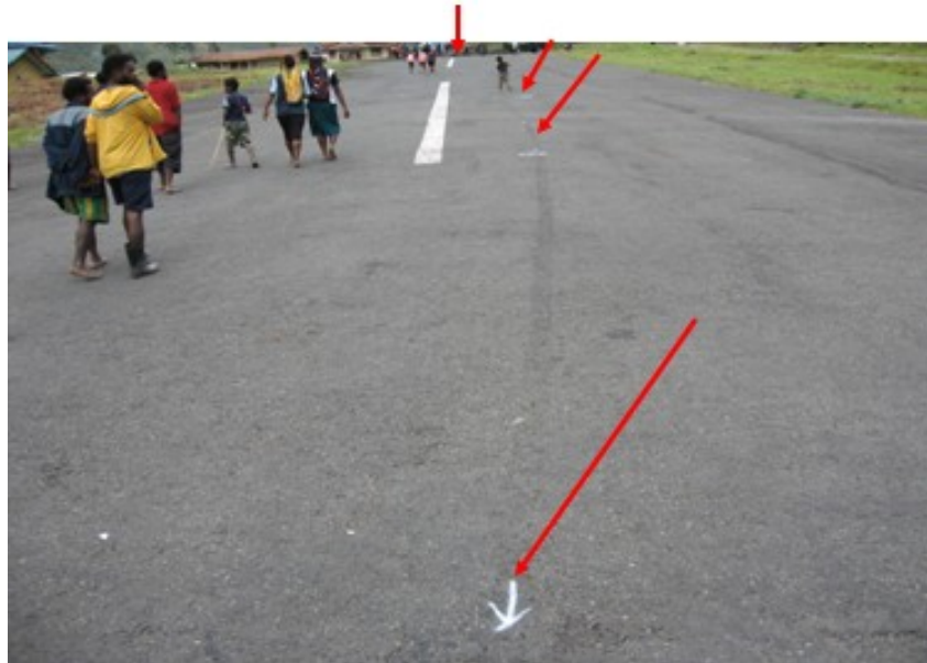
Figure 2 : View looking up slope back along the take-off track
