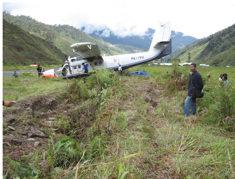
Figure 4 : The right shoulder of runway 27 showing rocks and ditch
