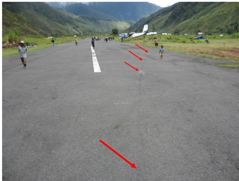
Figure 1: Left main wheel track showing runway excursion to the right
