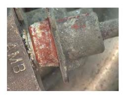
$\frac{\text{Figure 249:}}{\text{and diaphragm partially removed.}} \ \ \text{Remote ambient sensor, cover}$
